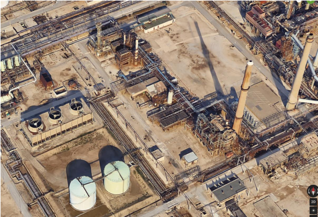
Figure 5 : View of the real site
