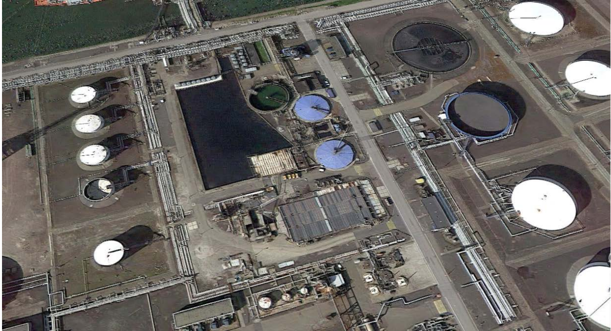
Figure 6 : View of the real site
