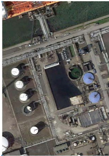
Figure 1 : views of Waste Water Treatment area
